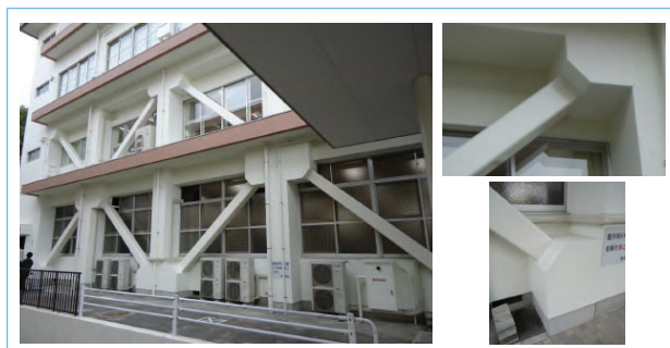
Development of low-cost seismic retrofitting technology by concrete filled steel tubular brace acting in compression for old buildings
