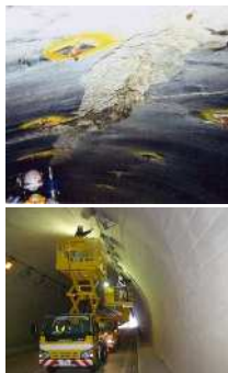
Inspection and diagnosis of tunnels
