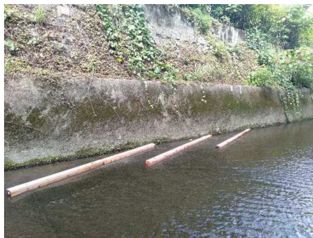
Waterfront environment restoration by barb structures
